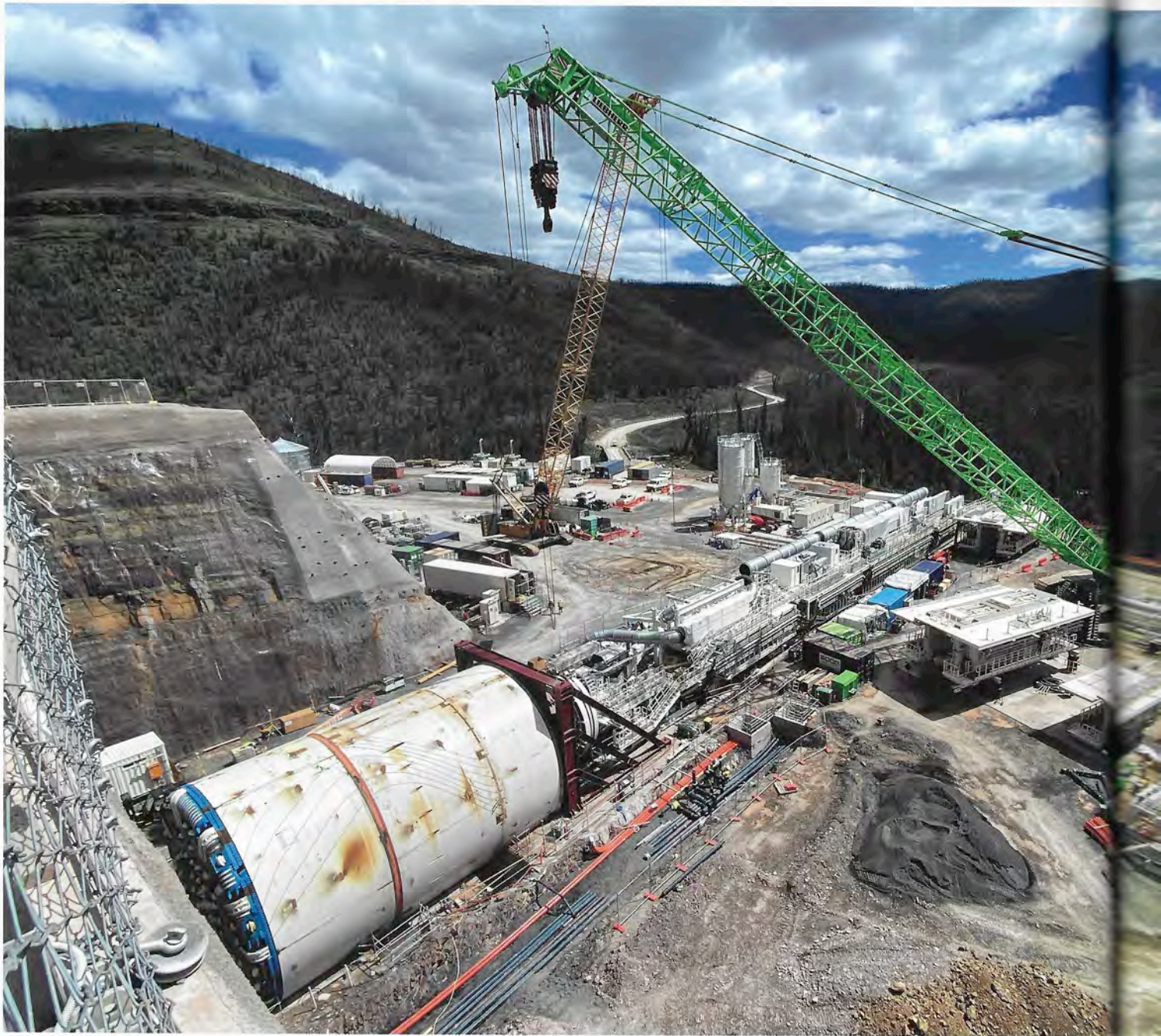
At 211 m long, "Kirsten" is one of the longest tunnel boring machines in existence. This is almost equivalent to the length of three Boeing 747s lined up in a row. At 3,350 tonnes it can accurately be described as a moving factory.
