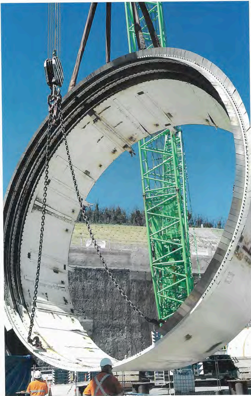
Lifting TBM "Kirsten" tailskin with 5,050 mm length and 94 tonnes weight. The 11,000 mm diameter of the tunnels is equivalent to a three-story building.
