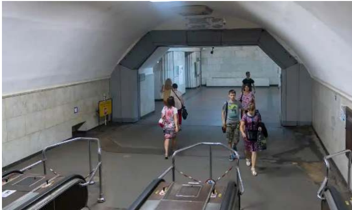
Arsenalna Station, Kyiv. A steel shutter can be lowered to seal off the tunnels and platform at the bottom of the escalators. Photograph: Bradley Garrett
