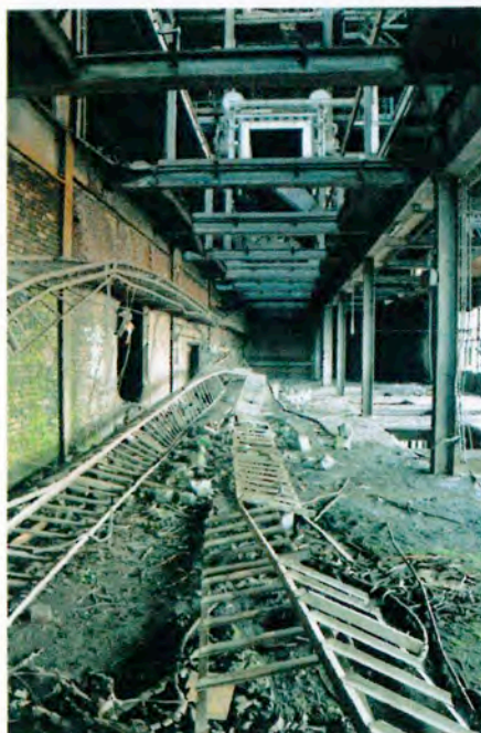
Figure 3.4. The twisted interior of Sinteranlage, Duisburg, Germany. Photograph by
